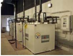
Generator day tanks are limited capacity tanks located adjacent to the generator set. The day tank provides a reservoir of fuel at atmospheric pressure to minimize the requirements on the generator engine fuel pump. Building codes typically restrict the capacity of day tanks within buildings especially above the lowest floor.
