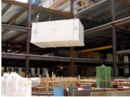
Bulk fuel storage tanks are typically located inside buildings in the lowest level. While local code requirements vary, the highest standard for the bulk fuel tank is a fire rated secondary containment tank. These tanks are available as horizontal cylindrical or rectangular units, with the rectangular units used inside buildings for space efficiency.
