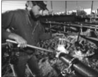
Fig. 5-3. Dualoy 3000/LCX can be tapered using the Ameron Taper Maker. The ratchet handle makes the Taper Maker convenient to use in confined spaces when repairing existing lines.
